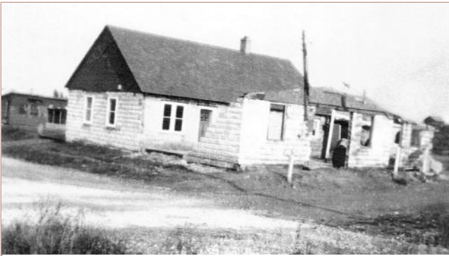
Pictured here is the Kitzinger family home that still stands on Waterford Avenue. At one time, the building housed the Shamrock Riding Academy. Photo shows part of the building being reduced to make room for the new road.
